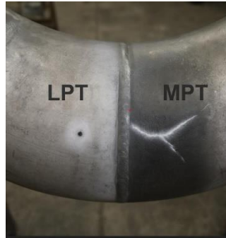
Gambar 7. hasil pengujian Liquid Penetrant Testing (LPT) dan Magnetic Particle Testing (MPT)
